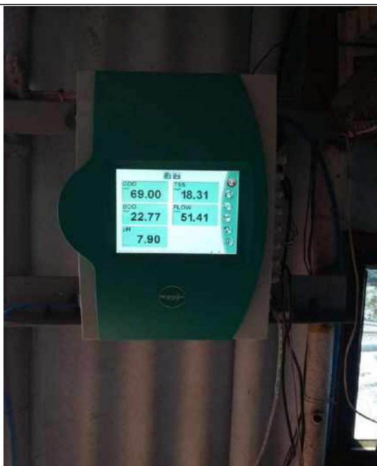
Online monitoring system for treated Effluent in Sugar ETP
