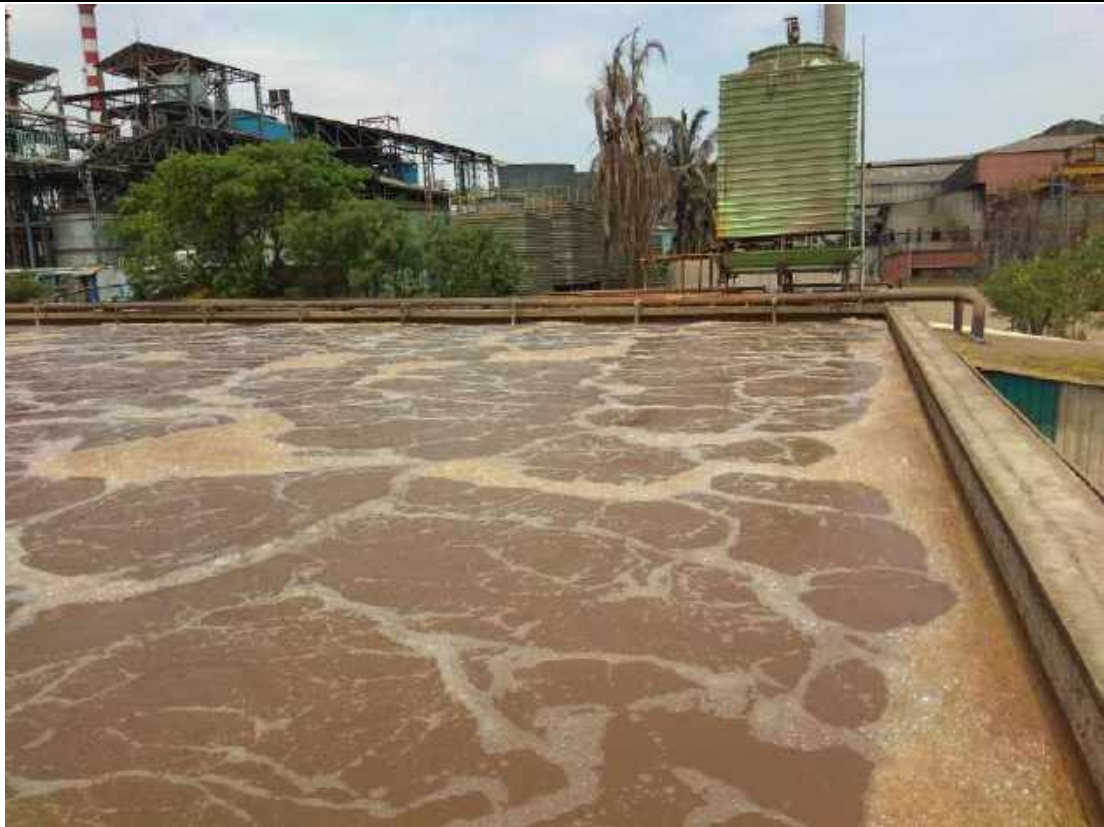
Polishing condensate unit (125m 3 /hr)
