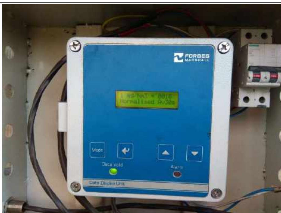
Installed Online Stack emission Monitoring System for 18 TPH boiler
