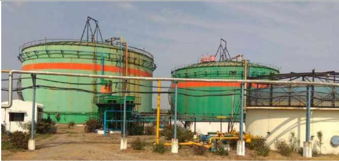
2 No's Of Bio-digester Plant (Capacity 450m 3 /Day Each)
