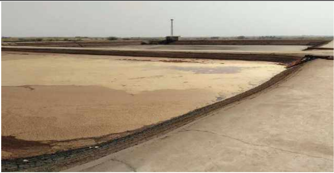
Impervious Lagoon storage for spent wash
