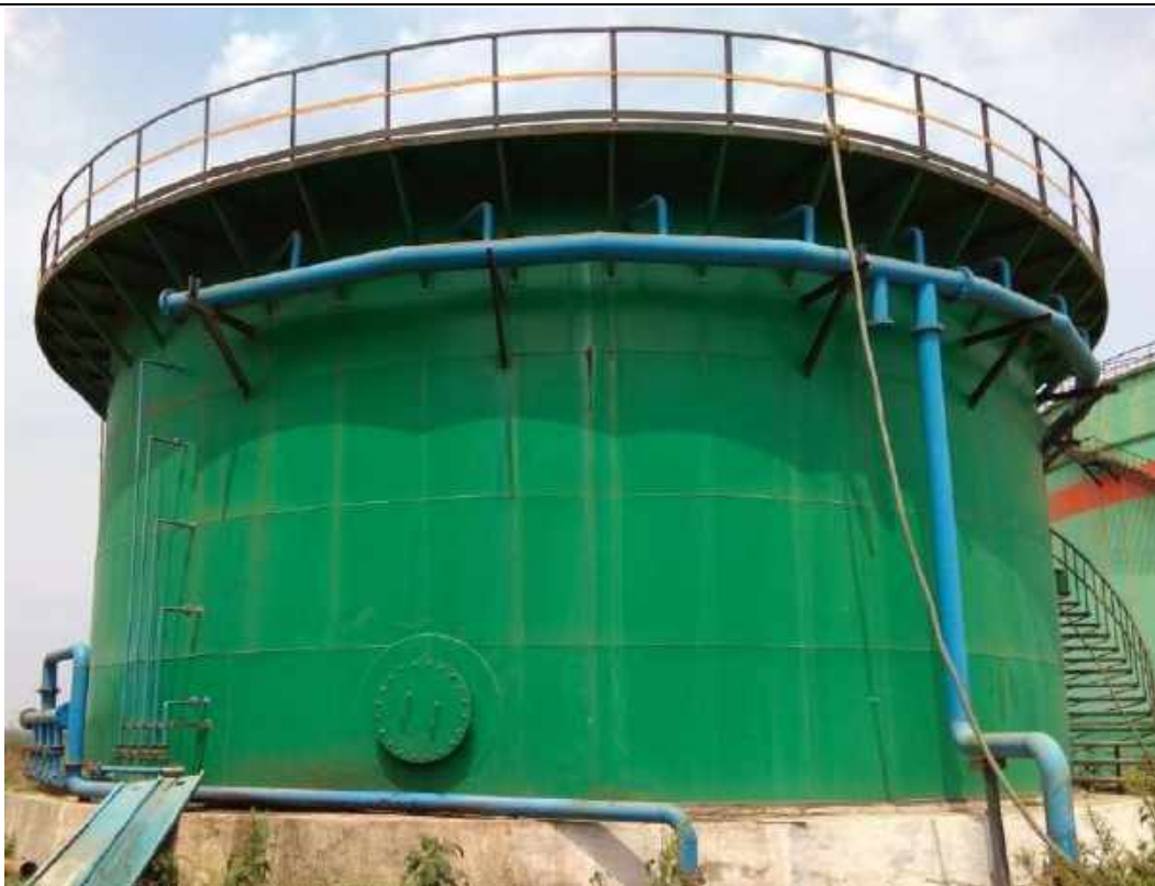
LESBAR reactor (capacity 1400 m 3 /day) for Expanded Sugar ETP
