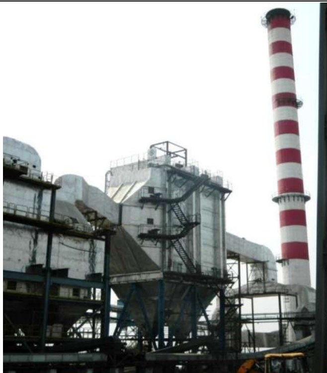
ESP for 130 TPH Boiler
