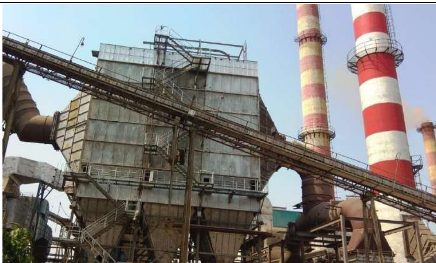
ESP for new 145 TPH boiler
