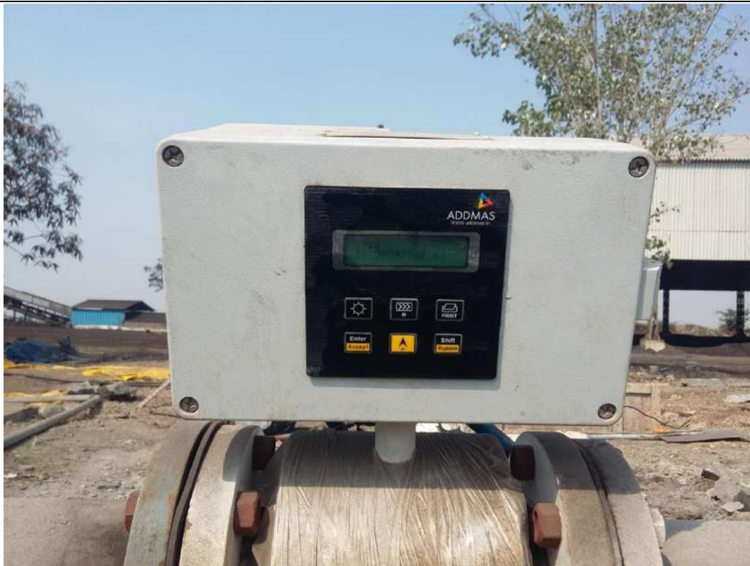
Flow meter installed for treated Effluent for Sugar ETP
