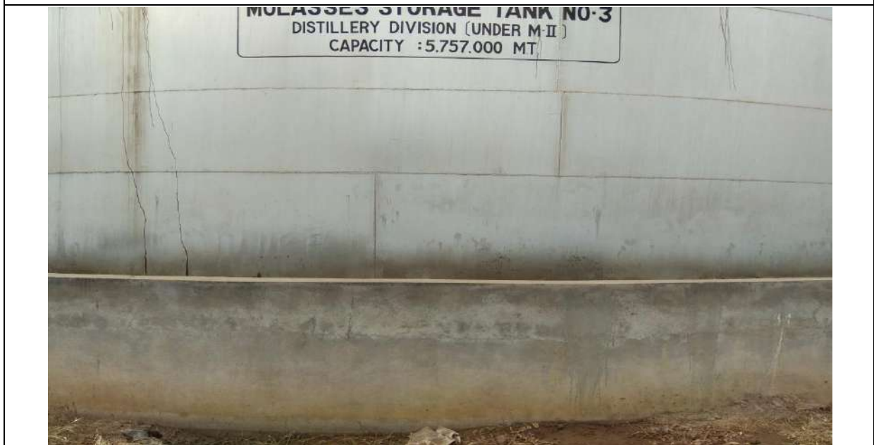
Dyke wall constructed around Molasses Tank
