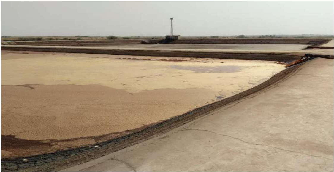
Impervious Lagoon storage for spent wash
