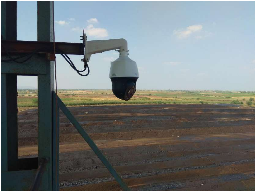
PTZ Camera installed compost yard site
